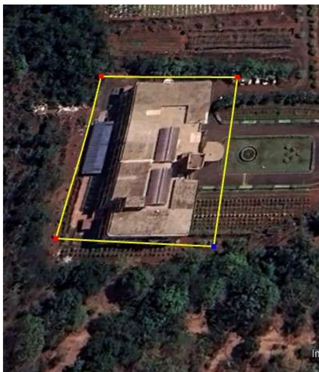
Figure 2. Main Building of DBSKKV
